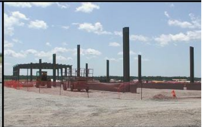
New Hangar Construction at Edenvale
